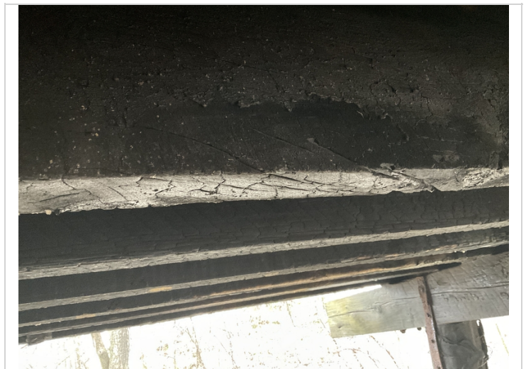
Span #3 girder #14 has diagonal crack across bottom face extending into girder three inches near center span.
