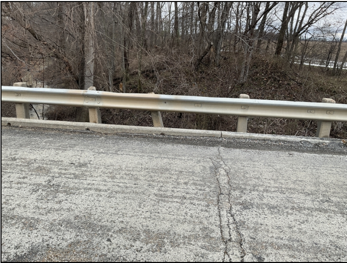
Span #2 first rail post not connected
