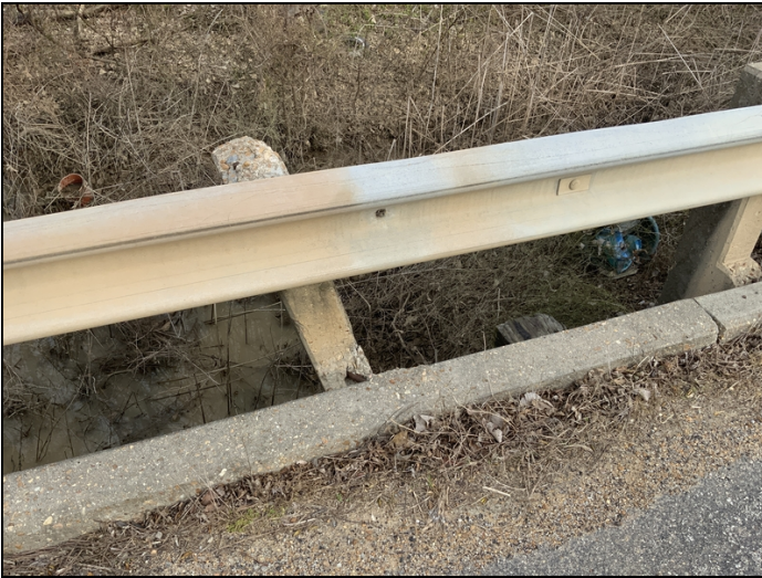
Typical missing rail post bolt.
