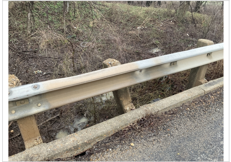
Span #2 right side, first rail post not connected.
