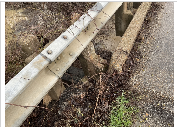
Span #3 right curb spalled 1' with exposed rebar with no section loss at abutment #2.
