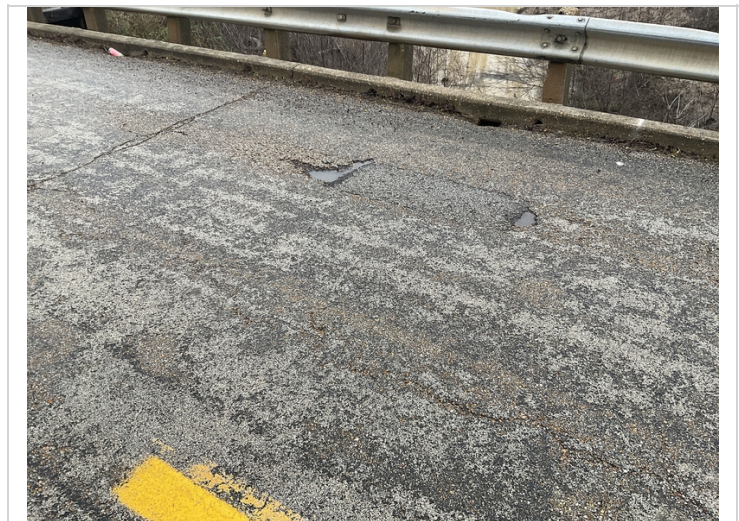
Span #2 right lane has a one foot spall in asphalt wearing surface that has been repaired and a two foot repaired spall in wearing surface. These repairs are being to fail with 2 small shallow spalls in repaired area.
