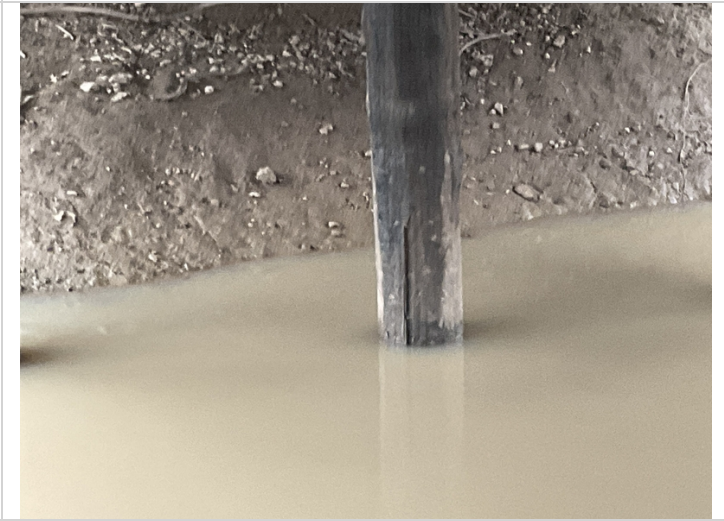
Bent #3 pile #3 has a moderate shake near bottom back side.
