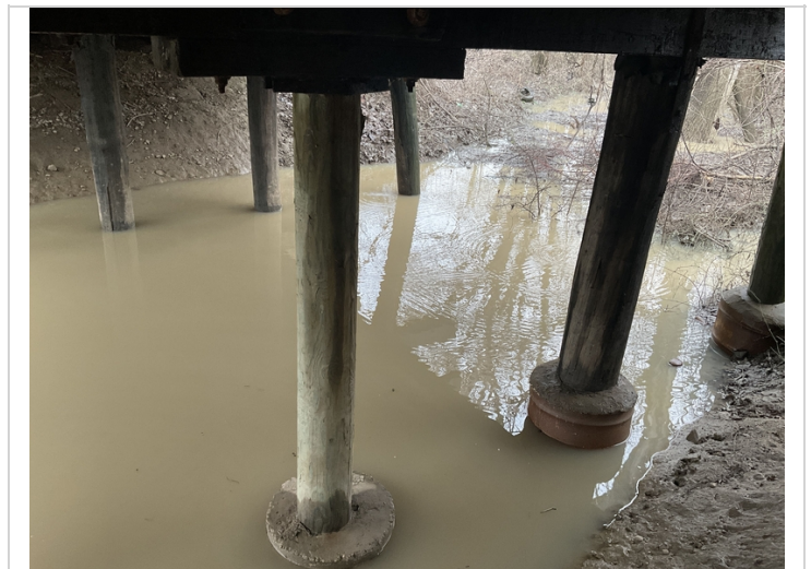
Typical spliced and encased piles
