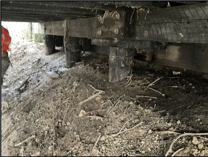
Bent #4 pile #3 has minor outer shell decay near ground approximately minor section loss.
