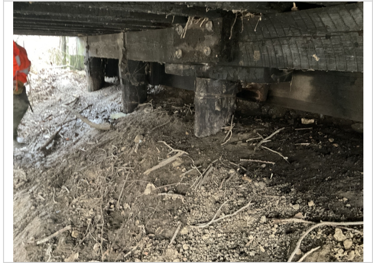
Bent #4 pile #3 has minor outer shell decay near ground approximately minor section loss.
