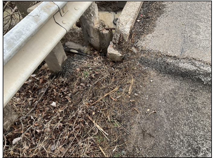
Erosion at abutment #2 right approach shoulder
