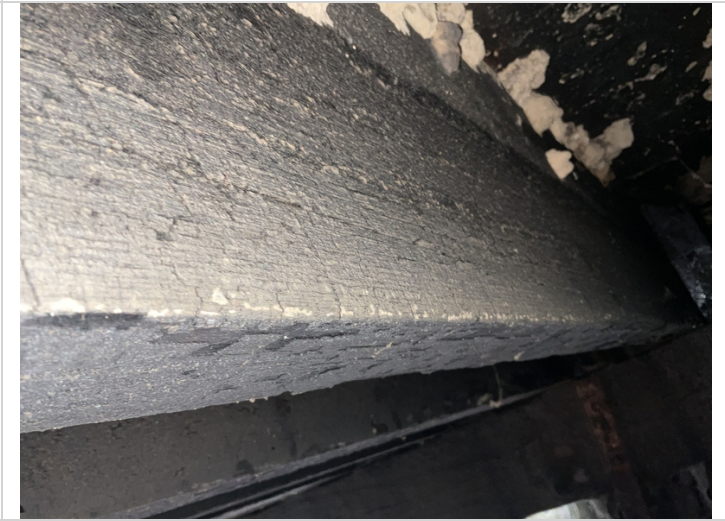
Typical girder fire damage
