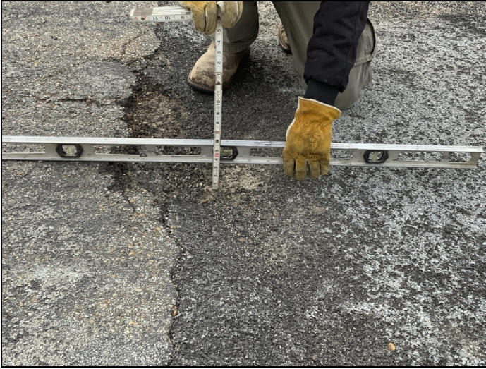
Abutment #2 approach roadway settlement.
