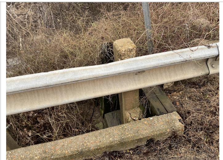
Span #3 left side, last rail post not connected.
