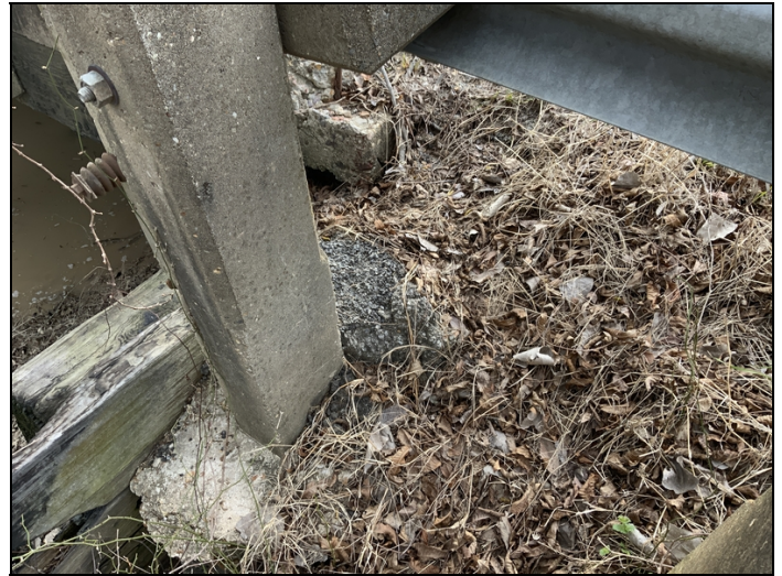
Erosion at abutment #2 right side.
