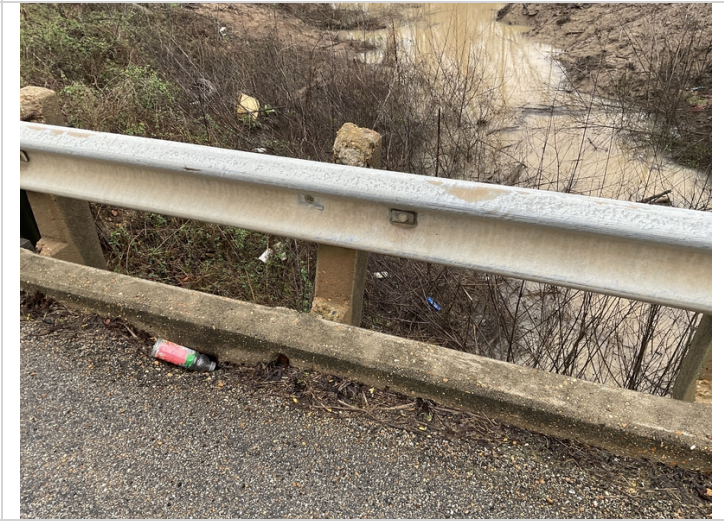
Span #1 left side, third post not connected.
