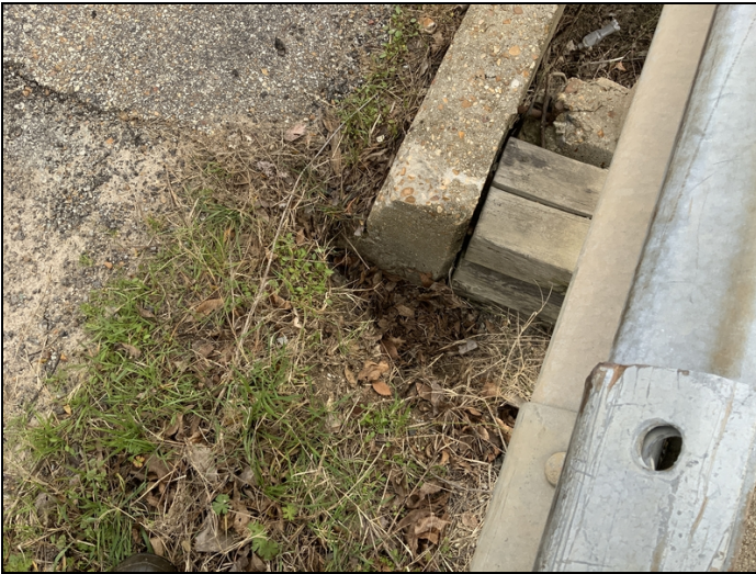
Erosion at abutment #2 left side.
