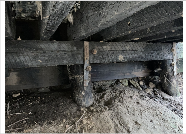
Typical abutment #2 cap
